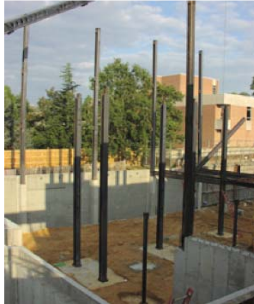
Figure 6.5.3- Steel Erection Started
