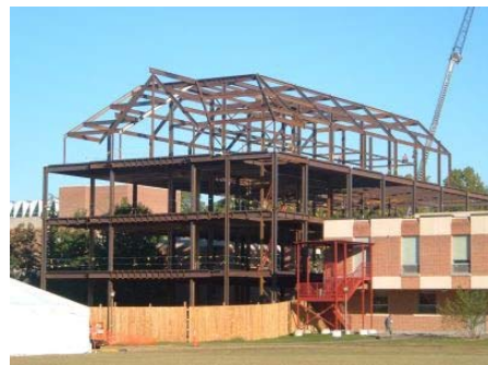
Figure 6.2.2 - Steel Framing
