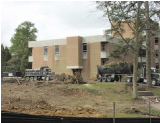
Figure 6.5.1- Preparation for Excavation
