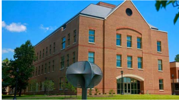
Figure 6.1.1 - Integrated Science Center North Facade
